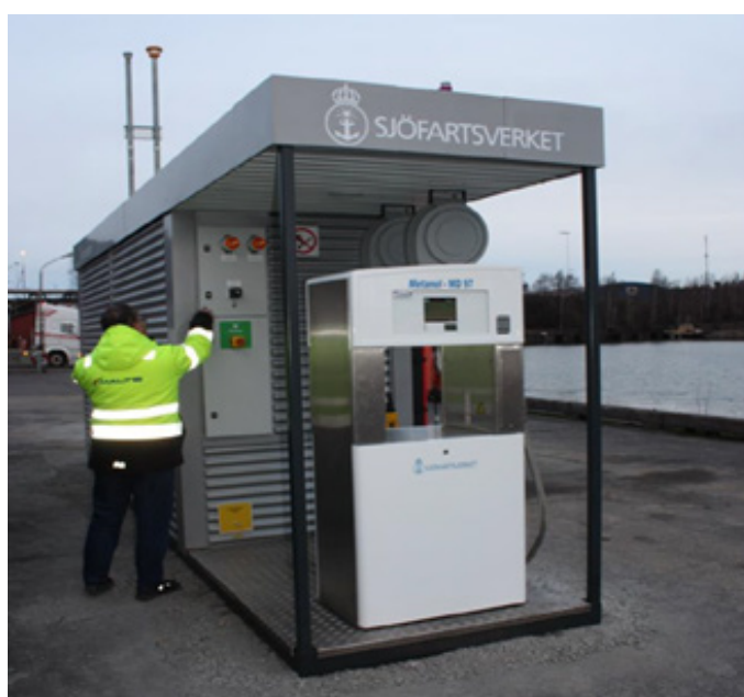
Figure 4 | Methanol (M97) refuelling facility at the Swedish Maritime Administration's Oxelösund pilot boat (Photo: J.Ellis) ( https://www.fastwater.eu/images/fastwater/news/FASTWATER_D71.pdf )
